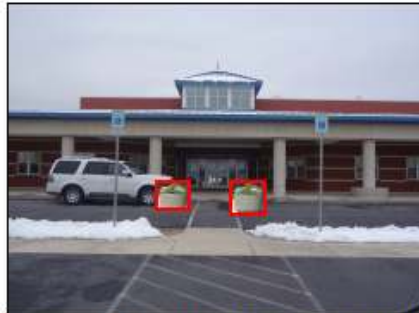
Photo 1: Vehicle impact bollards will prevent accidental or intentional vehicle strikes at the main entrance.
